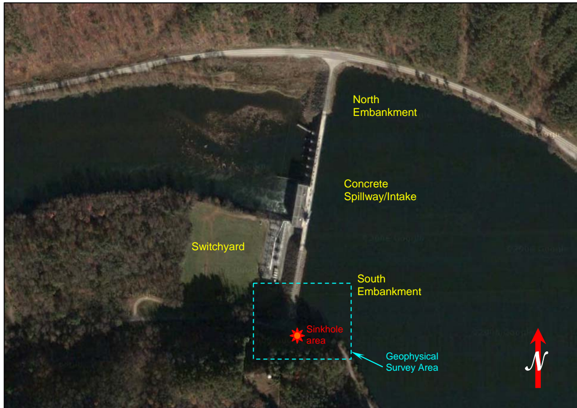
Figure 1. Aerial Photo of Chilhowee Dam Identifying Sinkhole Location and Geophysical Survey Location (Photo source: Google Maps)
